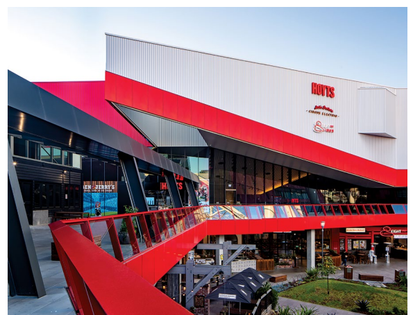
The Cinema Complex at District Docklands (Australia) uses welded beams and columns made from XLERPLATE® steel and roofing and cladding made from COLORBOND® steel. Both products have Environmental Product Declarations and a GreenRate™ 'Level A' rating.
